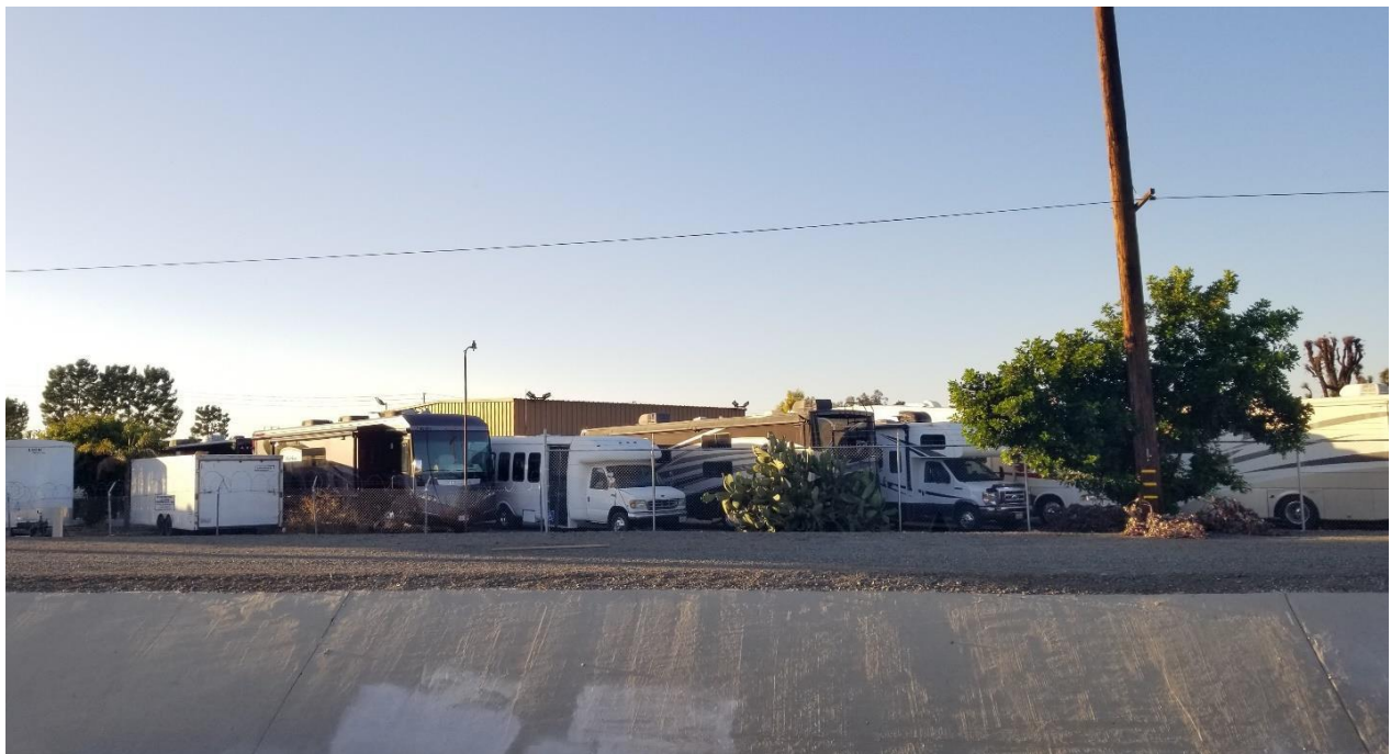
Figure 4: View of the project site looking north across the Anaheim-Barber Channel (in the foreground).
